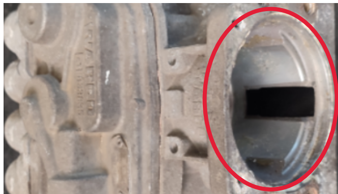
Dismantled device or missing components
