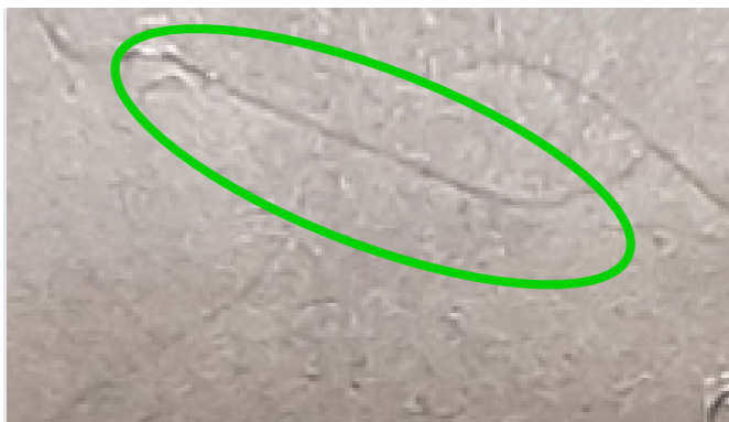
Scratches on external surface
