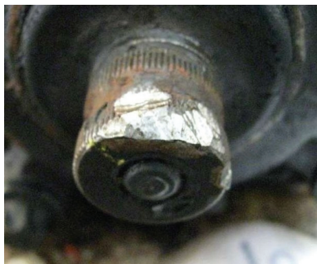
SHAFT DAMAGE (hammer)
